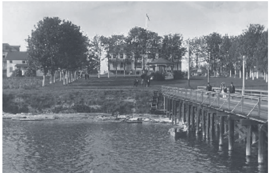
• Government-built Tulalip Indian School on the inner Tulalip Bay about 1912. The administration building is the only remaining structure.
